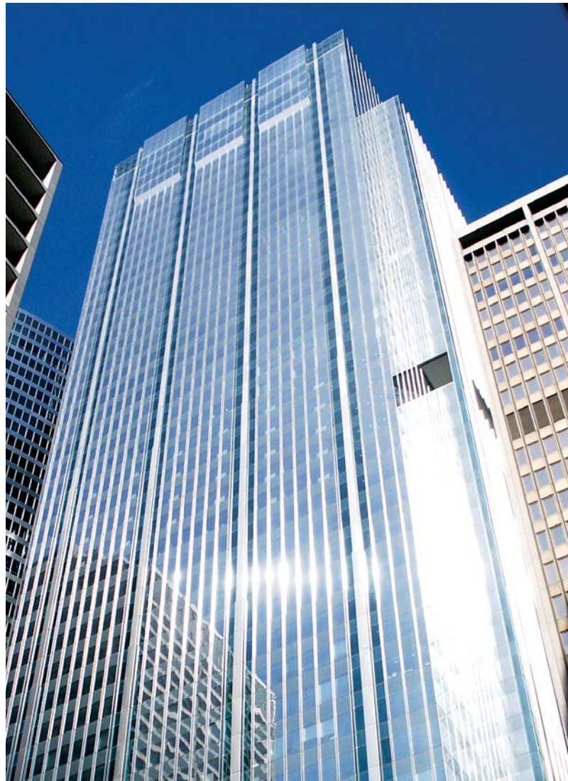
Thermafiber® Safing and FireSpan® mineral wool products provide the critical components of the perimeter fire containment system in the 111 South Wacker Building in Chicago, IL. Thermafiber® mineral wool insulation also contributed to the building's LEED® Gold Rating.
