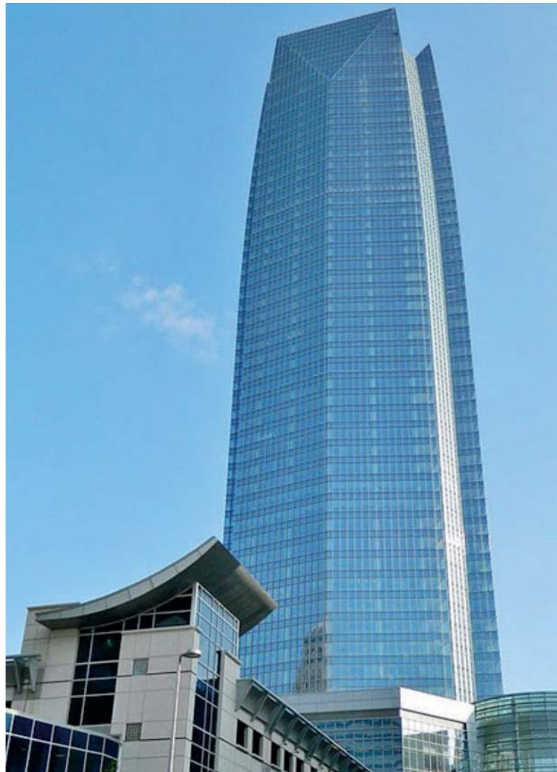
Thermafiber® mineral wool insulation was used in the perimeter fire containment system in the Devon Energy Center in Oklahoma City, OK.
