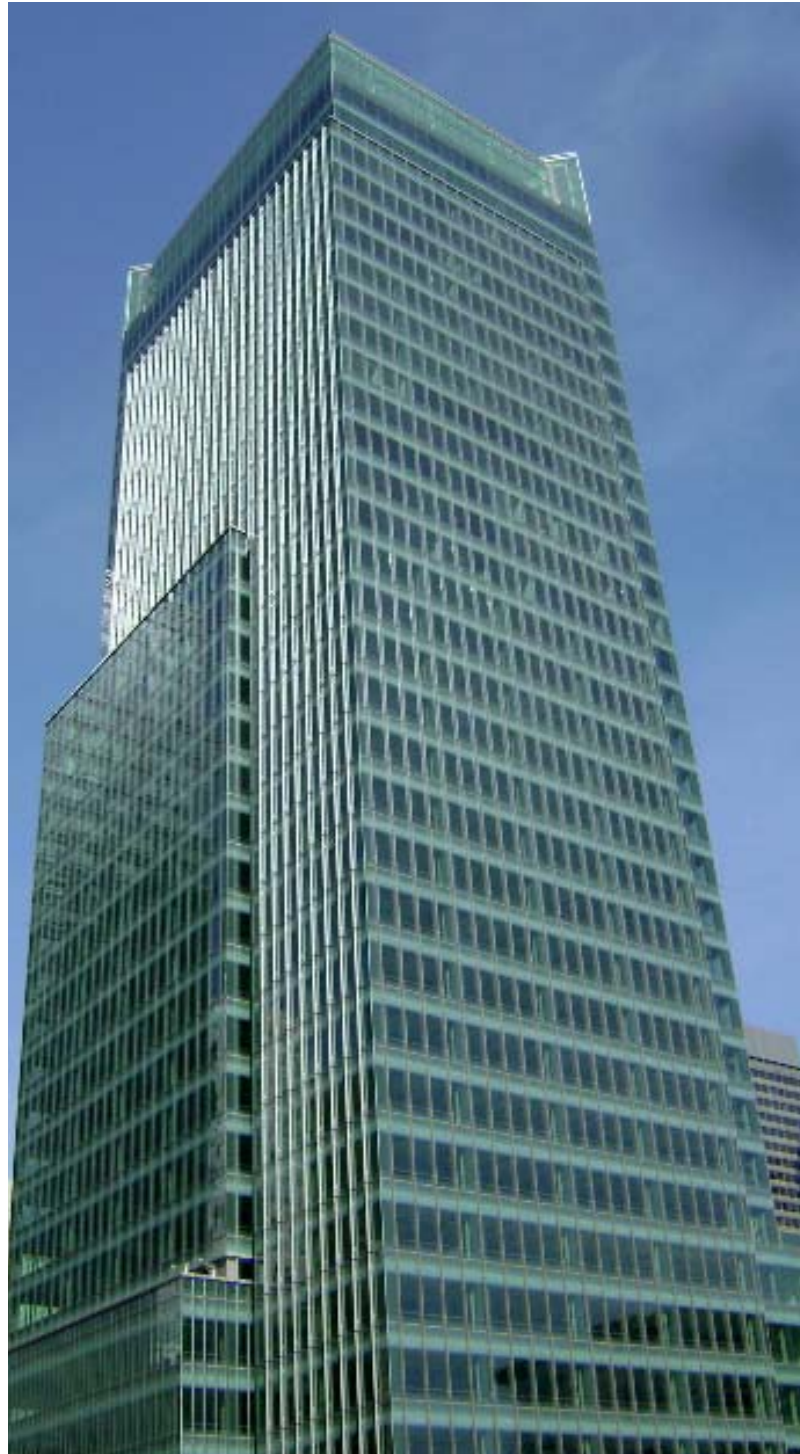
Thermafiber® Impasse® Hangers were used to secure the Firespan® mineral wool insulation for the perimeter fire containment system in the 555 Mission building in San Francisco, CA. Thermafiber® insulation also contributed to the LEED® silver rating for this building.
