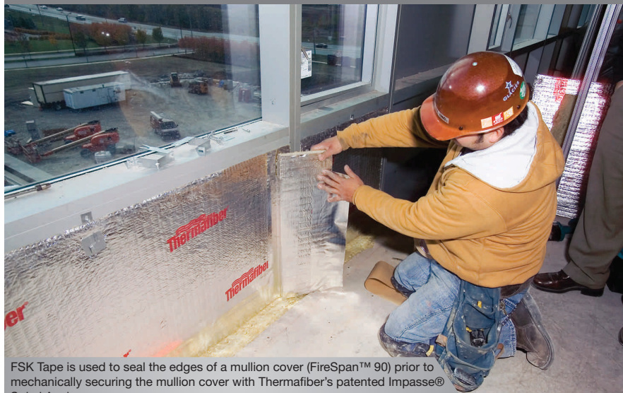
Aluminum Foil and FSK Tapes are used in curtain wall buildings like these in New York City. The tapes work in conjunction with foil faced FireSpan™ Curtain Wall Insulation to create a vapor barrier for the building envelope.
